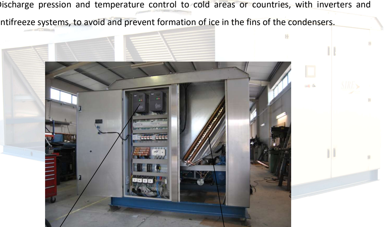
Fans speed inverter, to control the pressure on condensers
