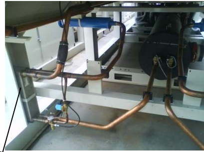
Economizer, increase 15% of capacity, with less energy (optional)
